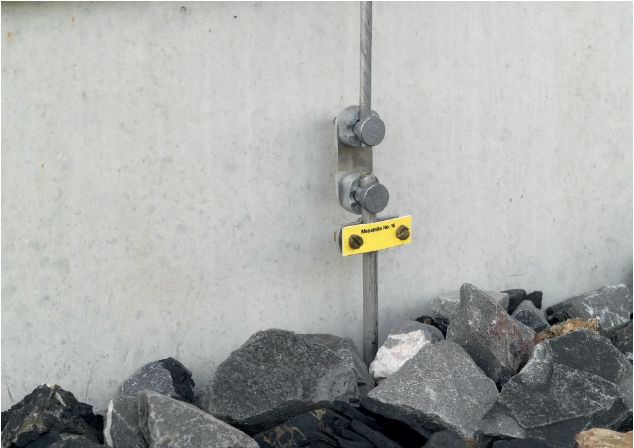
Separation point on a metal facade
