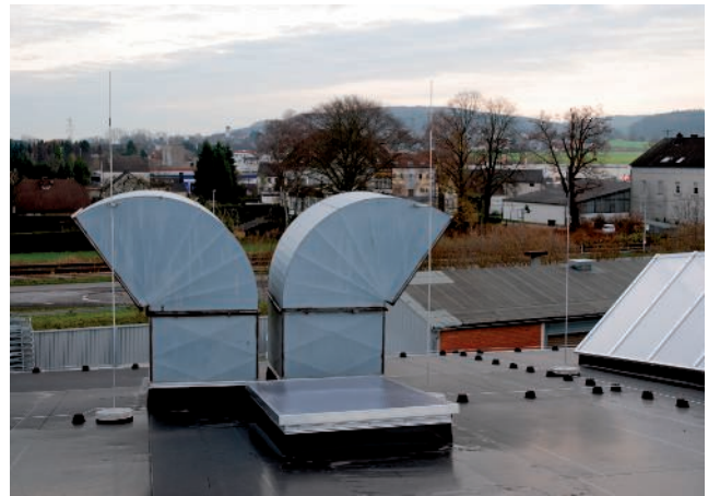
Isolated system with GRP holders
