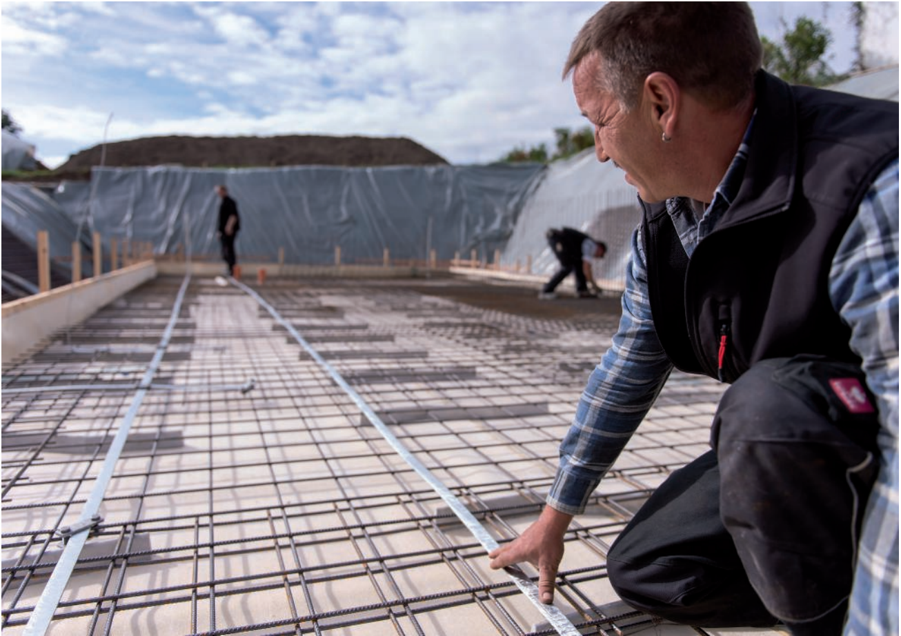
Installing a foundation earth electrode
