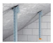
Variable head plate with US 3 support Installation of the variable head plate, type KU 3 V on US 3 support.
