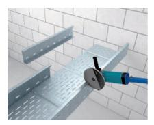
Creation of a tee with add-on corner Removal of the side rails from the wide span tray.
