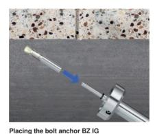
The Wedge Anchor BZ-IG is placed on the setting tool BZ-IGS. It must be ensured that the thread size of the setting tool fits to the corresponding anchor bolt.
