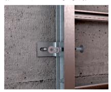
Fastening of industrial vertical ladder Industrial vertical ladders are fastened to steel girders using mounting angle, type BW80/55.
