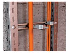
**Cable fastening with U clamp** Fastening of a cable to the rung with U clamp.
