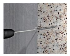
**Cleaning with steel wire brush** The cleaning process with blow and brush must be carried out twice.
