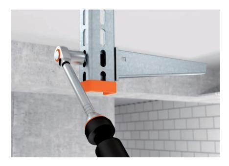
Different tightening torques apply when mounting a cable support system. Please note that the specified torques are only intended as rough, non-binding guide values. (See VDI 2230)!
