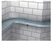
Installation of bend (width 400 – 600 mm) The bend in widths 400 to 600 mm is connected to the cable tray using connectors and a joint plate. Additional supports should be planned for the area of the fittings.
