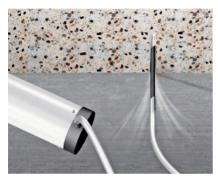
Blowing out of the drill hole Freeing the drill hole of dust by blowing it out.
