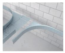
**Creation of a tee with add-on corner** Installation of the second add-on corner, type WEAS 110.
