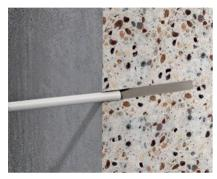
Application of the injection mortar Pressing the injection mortar into the hole
