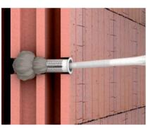
Applying the injection mortar
