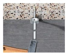
Hammering the bolt anchor BZ IG Hammering the bolt anchor BZ-IG with the appropriate setting tool. Subsequently, the component to be mounted can be secured.
