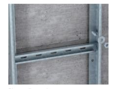
**Direct wall mounting** Direct fastening of the vertical ladders LG and SSL with anchor bolts on the wall.
