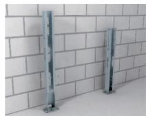
Installation of motor connection column with column foot
