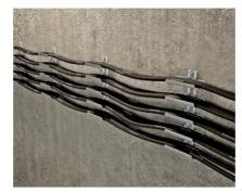
Factory pre-assembled cable carrier trays help in a fast installation.
