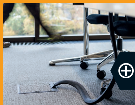
Device inserts supply workplaces and other points in the middle of rooms with power and data connections above the floor.
