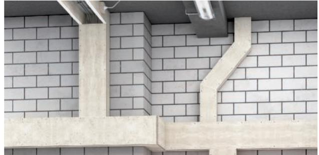
Mounted fire protection duct on wall and ceiling
